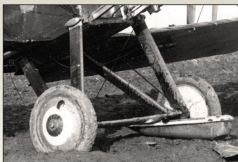
Early steel undercarriage with wooden fairings from the same aircraft seen on page 27. Note the fabric strips wrapped around the struts and fairings to bind them together. Undercarriage struts of this type were usually doped in PC10.
